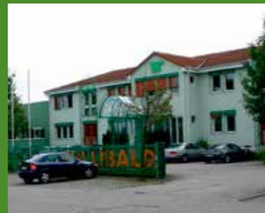
Part of the company headquarters in Sentenhart
