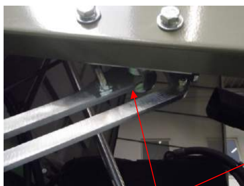
Bolt is engage in the hood securing.
